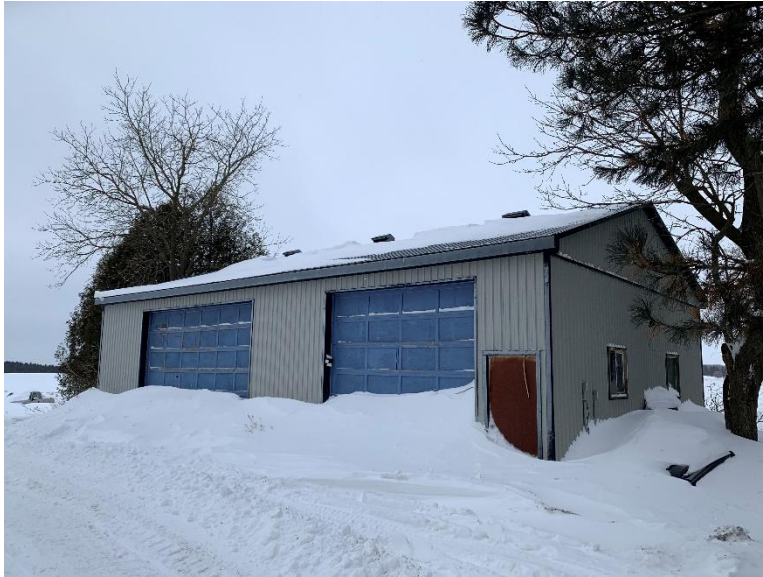
Figure 17: Garage to the west of the residence, looking northwest (A.S.I., 2025)
