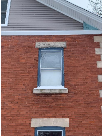
Figure 15: Lintel and sill on the east elevation (A.S.I., 2025)
