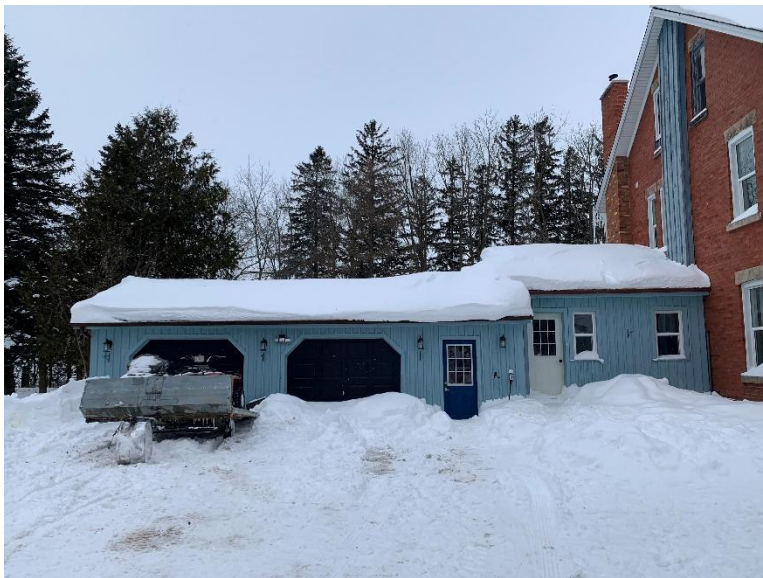
Figure 16: Addition on west elevation, looking north (A.S.I., 2025)
