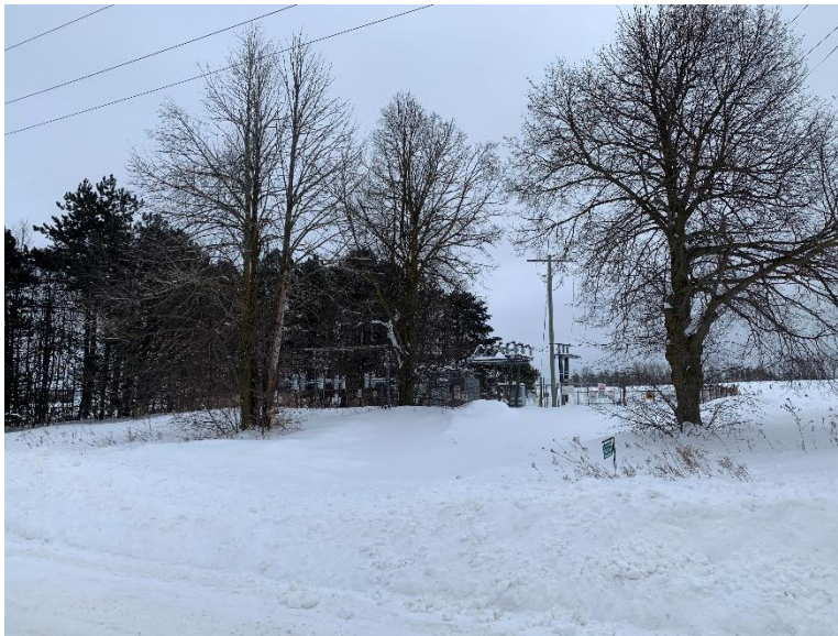
Figure 34: Electrical facility surrounded by trees on south side of Sideroad 27 (A.S.I., 2025)
